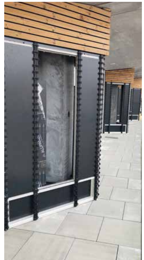
Elegant construction in Aarhus harbour - The plastic used in large projects is not always visible. In the Bjarke Ingels building Ø4 in Aarhus harbour, fire-resistant aluminium sandwich sheets were used to line ventilation triangles. For this project we delivered 75 different cut to measure types of plastic sheets.
