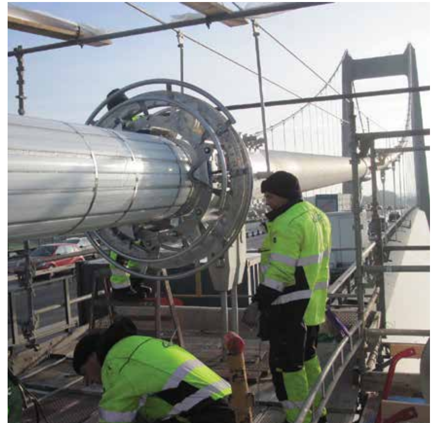
Processed PE-HD rails that are mounted on the fire damaged wire on the new Little Belt Bridge
